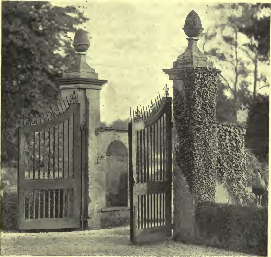
FIG. 5. WOODEN GATES WITH IRON BARS AND CRESTING AT GROOMBRIDGE PLACE, KENT. LATER XVIIITH CENTURY.
