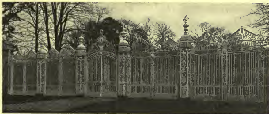
FIG. 22A. THE SCREEN AT LEESWOOD HALL.
