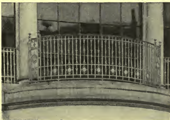
FIG. 104. BALCONY TO FIRST FLOOR WINDOW, BOODLES CLUB, ST. JAMES'S STREET.
