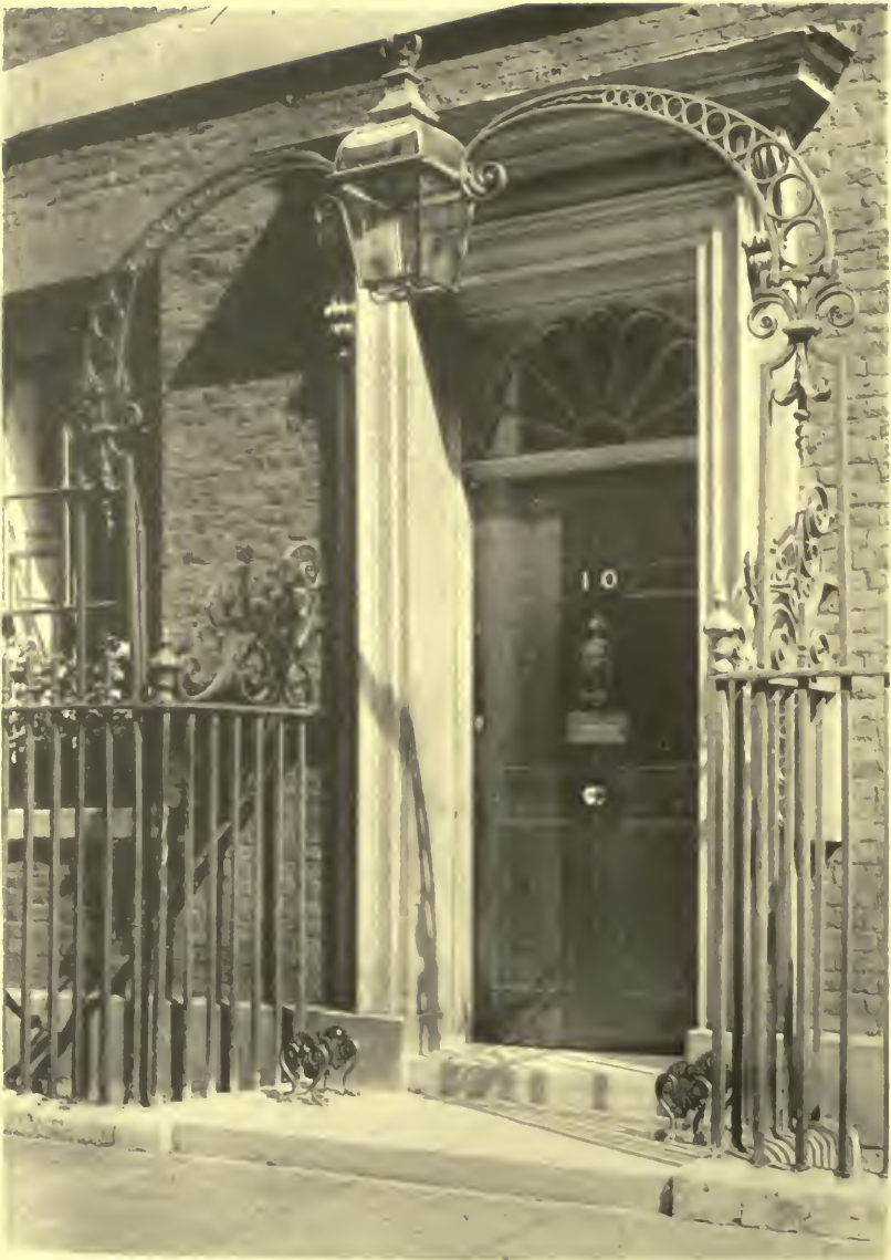
ARCHING LAMP HOLDER AND RAILINGS, 10 DOWNING STREET.
