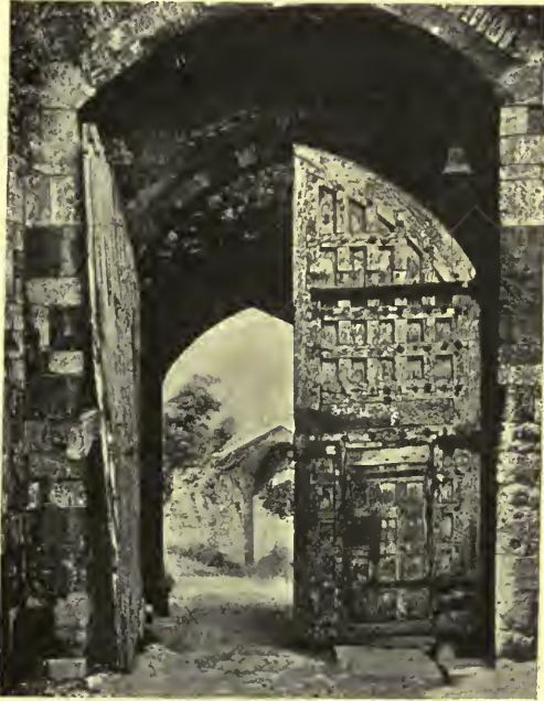
FIG. I. THE CASTLE GATE, CARISBROOKE, GUARDED BY A PORTCULLIS.
