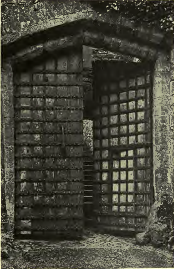
FIG. 3. DOORS TO DUNSTER CASTLE, SOMERSET.
