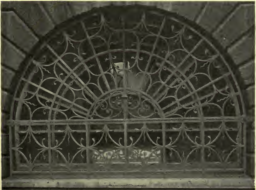
FIG. 107. PROTECTIVE GRILLE AT THE MANSION HOUSE.
